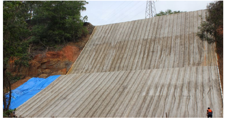
Figure 2. Typical Type I GCCM slope protection application.
