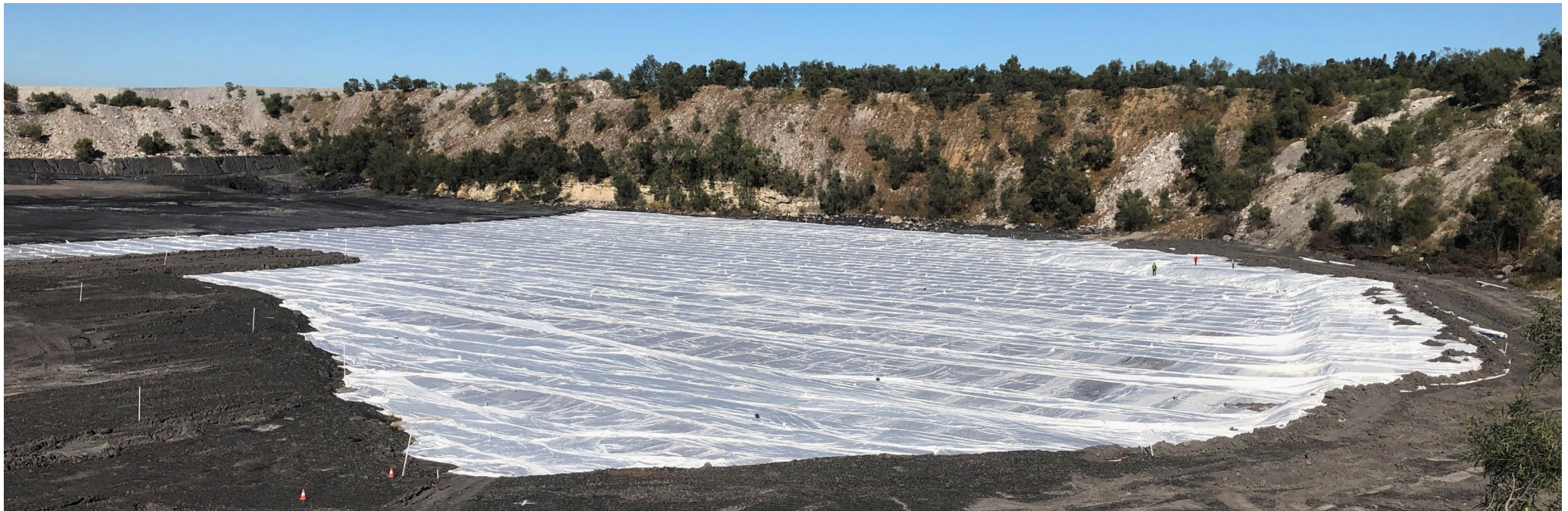
Infilling between parallel fill fingers to complete fill closure
