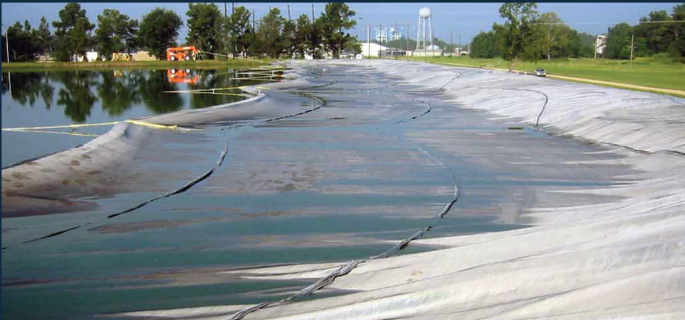
Pulling MIRAFI geotextile reinforcement panel across surface of sludge pond
