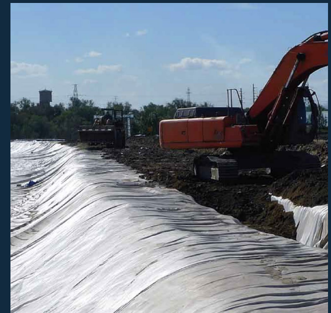
Anchorage of MIRAFI geotextile panel around periphery of sludge pond
