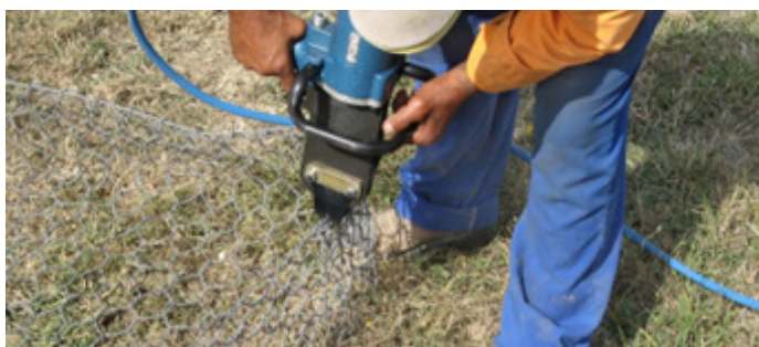
Fig. 6 – Pneumatic lacing tool
