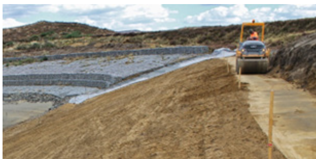
Fig. 3 – Prepared foundation
