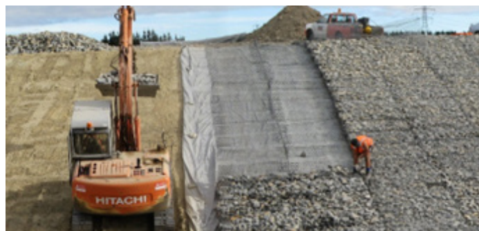
Fig. 10 – Filling from bottom cells
