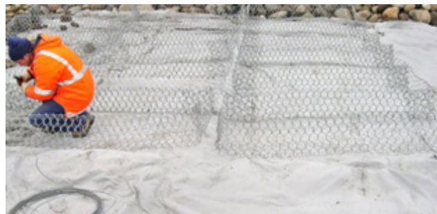
Fig. 4 – Prepared foundation
