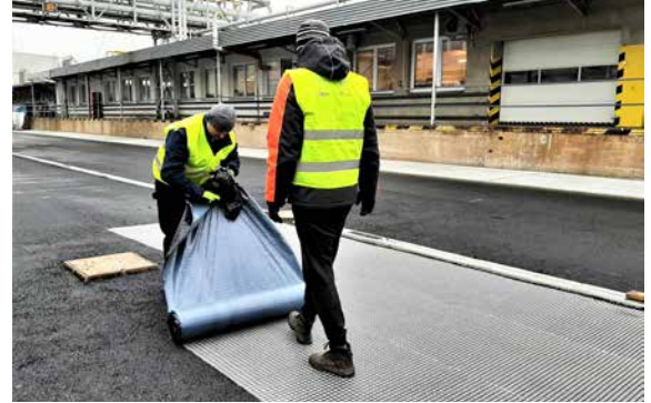
Pic. 4: ADFORS GlasGrid Rapid instalation
