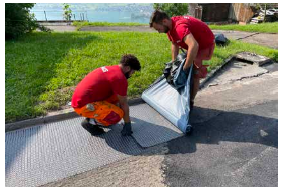
Pic. 2: ADFORS GlasGrid Rapid application for local repairs
