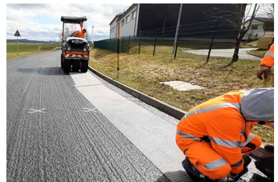
Pic. 3: ADFORS GlasGrid Rapid installation and adhesive layer activation
