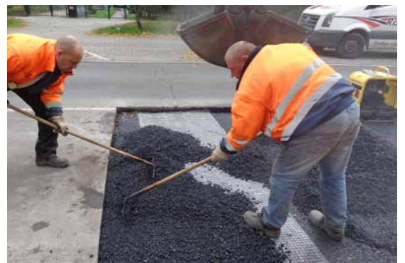
Pic. 18: HMA application over ADFORS GlasGrid Rapid
