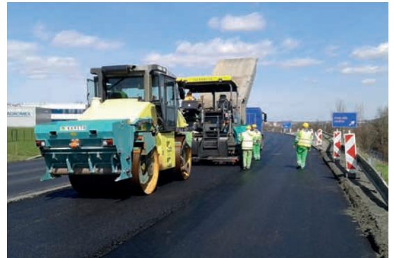
Pic. 9: Pave Overlay
