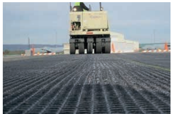
Pic. 2: Typical installation and glue activation on a levelling course
