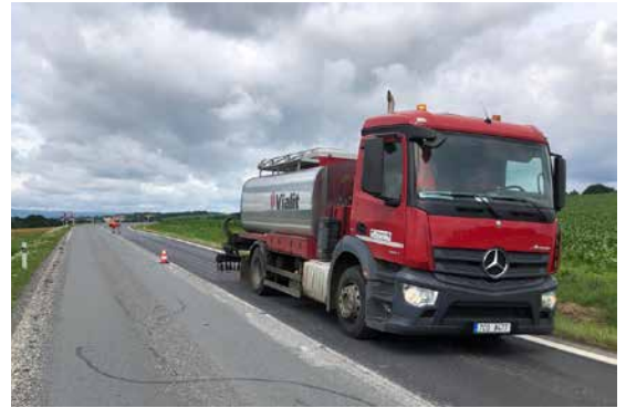
Pic. 8: Tack coat application over ADFORS GlasGrid GG
