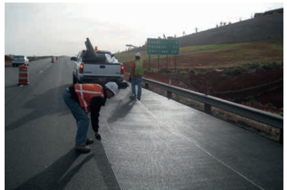
Pic. 4: Manual Installation of ADFORS GlasGrid
