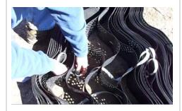
Figure 17 Threading Tendon and Attaching ATRA Tendon Clips
