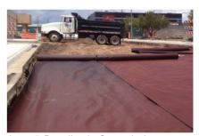
Image 7. Extending the Geosynthetic Reinforcement up a Vertical Face
