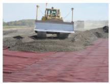
Image 4. Spreading aggregate over geosynthetic
