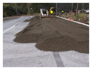
This solution saved time and money. The site was secured, quickly and efficiently, by using the laminate. Another advantage was that the site was not held up due to bad weather. A rain event when the subgrade was open would have delayed the construction by weeks to allow the site to dry out. Using the Tensar Laminate meant that the site construction could continue quickly.
