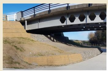
Completed Green Terramesh structure with both vegetation and rock face.
