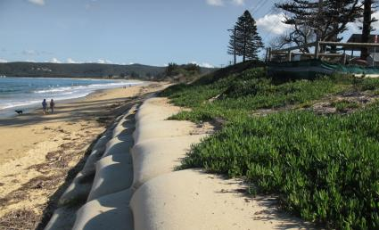
Following advice from coastal engineering experts, we decided that installing these sandbags, under emergency works, was the best way to quickly and effectively stabilise the sea wall and shield the local road.
