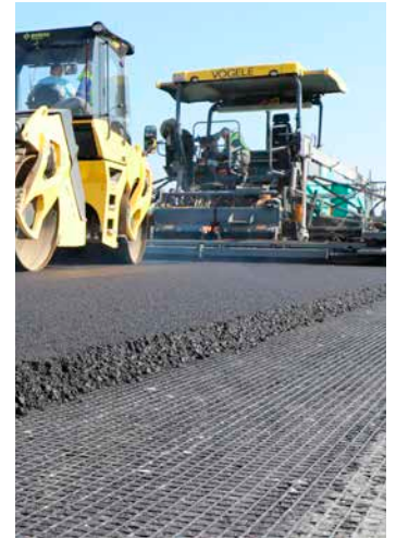
Installation of ADFORS GlasGrid at Atatürk Airport, 2010
