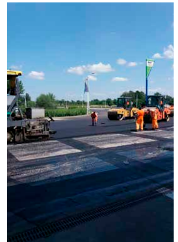
Installation of ADFORS GlasGrid Rapid in Belgrade, 2018
