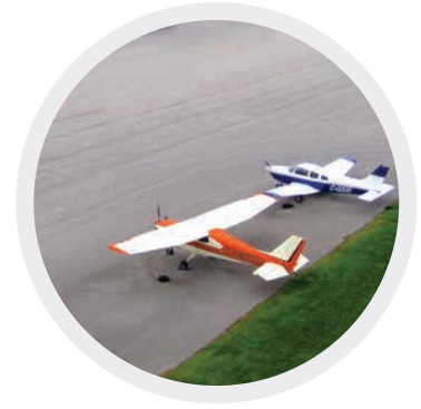
State of the pavement after 20 years in service (photo May 2012)
