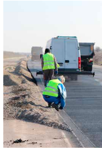
Installation of ADFORS GlasGrid at Atatürk Airport, 2010
