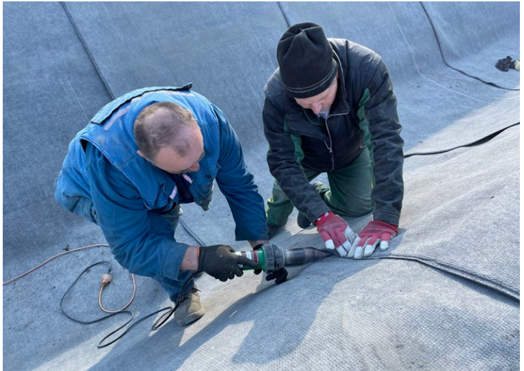
CCX-M™ overlapped by 100mm and thermally bonded together
