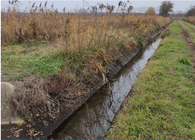
Existing canal with vegetation and precast concrete slabs
