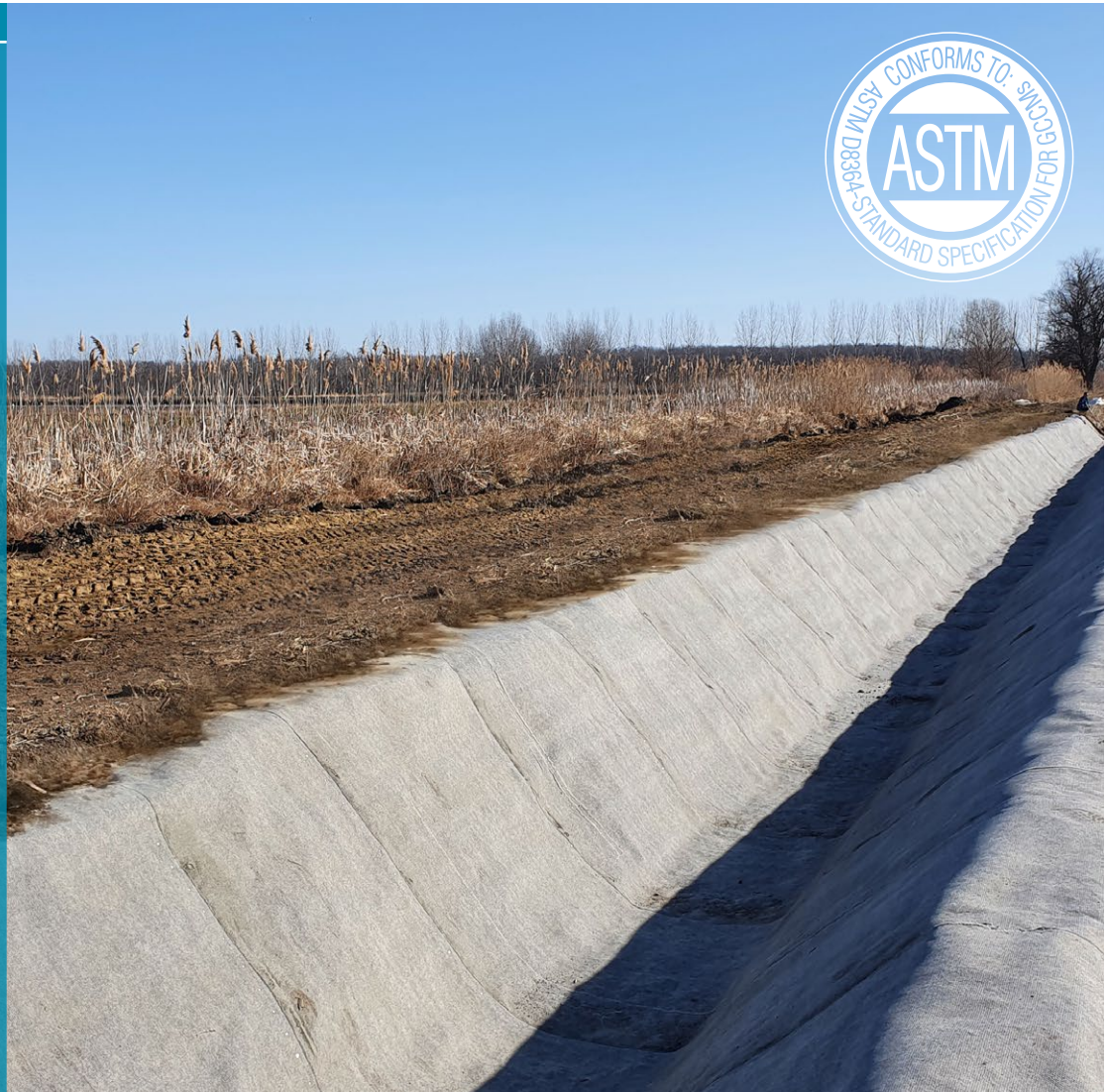
Completed CCX-M™ installation
