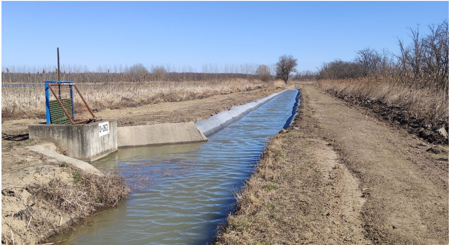
Completed CCX-M™ Installation in full operation
