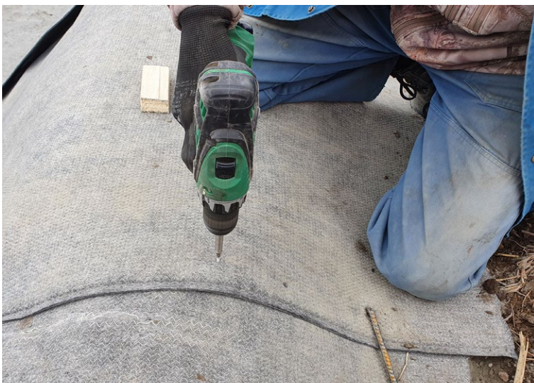
CCX-M™ overlaps secured with 30mm stainless steel screws
