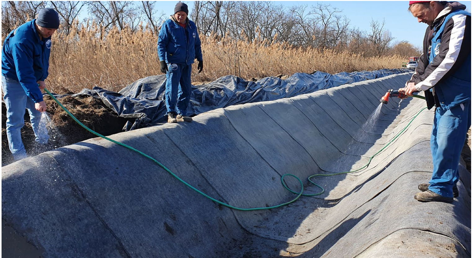
CCX-M™ hydrated on each side of the canal
