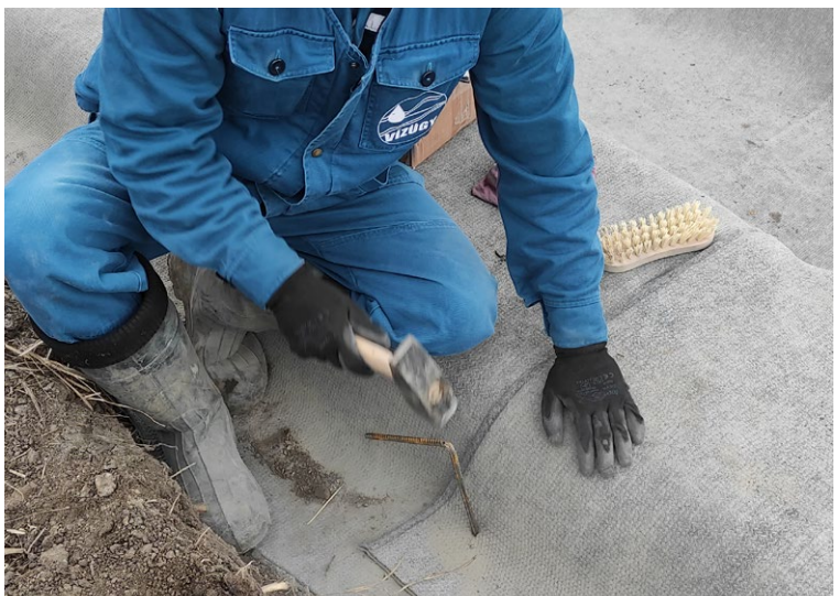
CCX-M™ pegged in the anchor trench
