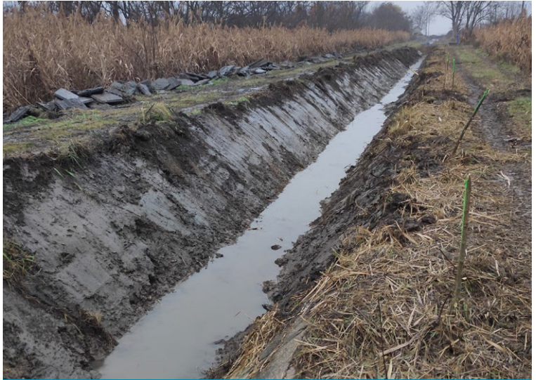
Precast concrete slabs removed and canal reprofiled
