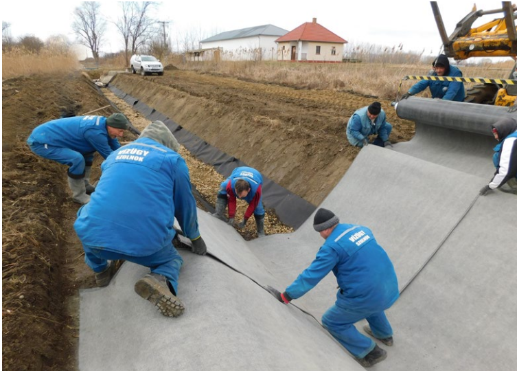
CCX-M™ laid transversely with aid of an excavator and spreader beam
