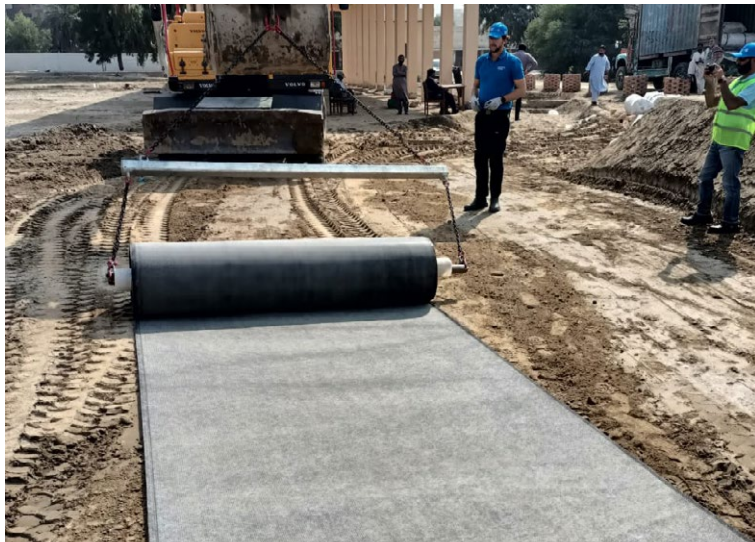
CCX-B™ deployed with the aid of an excavator and spreader frame
