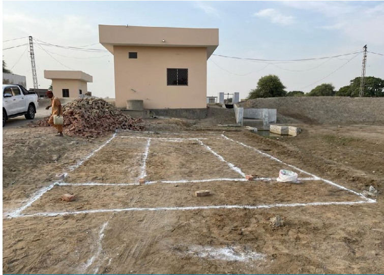
Planned pond works before installation
