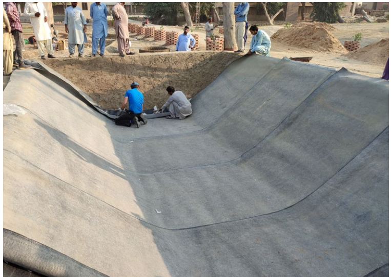
CCX-B™ laid transversely and anchored
