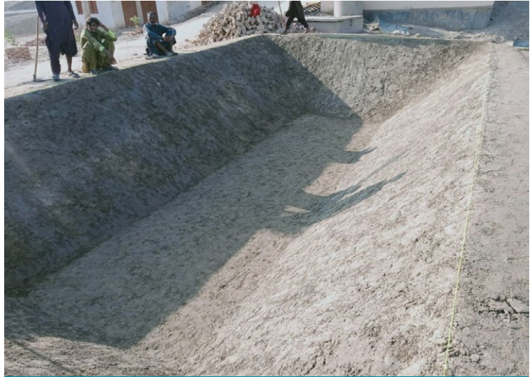
Completed pond earthworks
