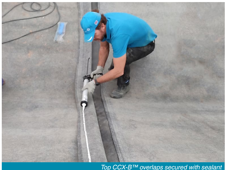
CCX-B™ laid transversely and anchored
