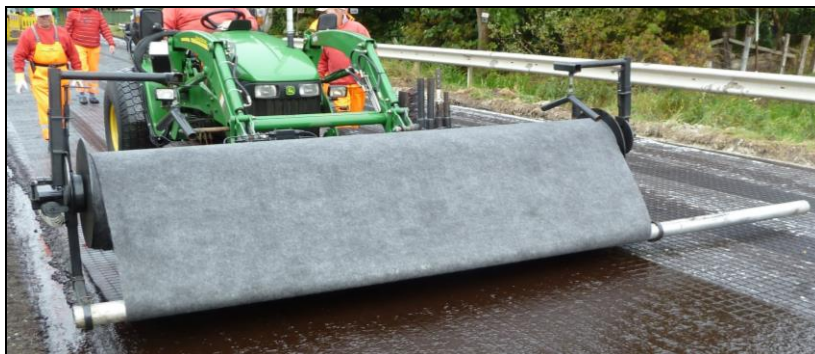
Picture 5: Grid Installation machine
