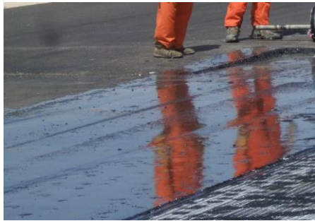
Picture 2: Mirror effect of fresh bond coat/black prints on product
