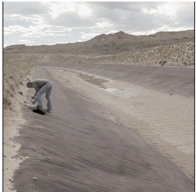
The main canal of the Casper-Alcova Irrigation District, more than ten years after installation of the Teranap Geomembrane.
