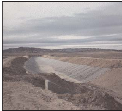
Installation of Teranap Geomembrane in the main canal of the Casper-Alcova Irrigation District in 1991.
