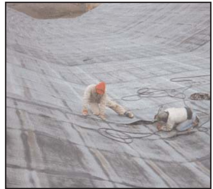
Installation of Teranap Geomembrane in the main canal of the Casper-Alcova Irrigation District in 1991.
