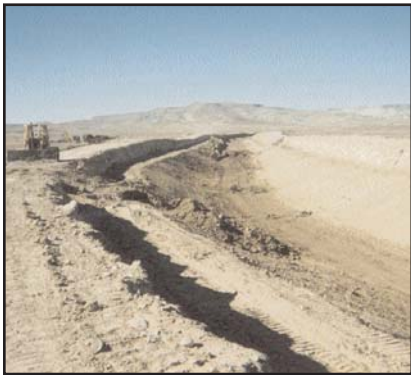
Installation of Teranap Geomembrane in the main canal of the Casper-Alcova Irrigation District in 1991.
