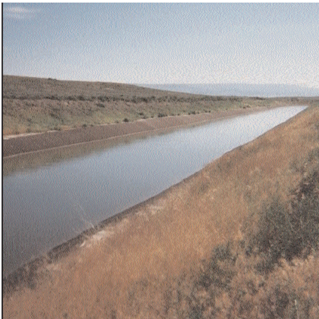
The main canal of the Casper-Alcova Irrigation District, more than ten years after installation of the Teranap Geomembrane.
