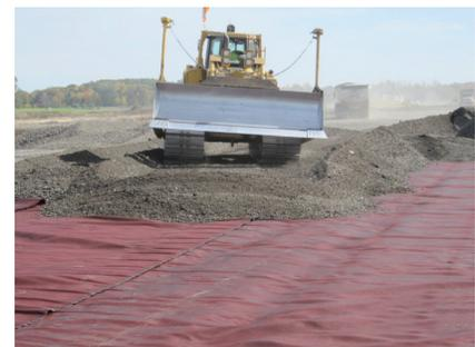
Image 4. Spreading aggregate over geosynthetic
