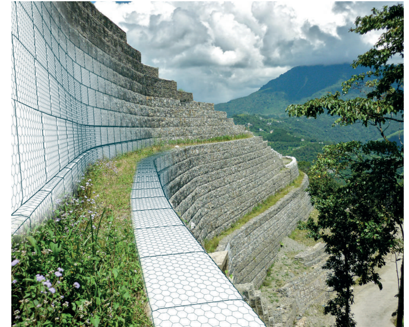
MacSTARS enabled the design of high-end and challenging structures in the most diverse conditions
