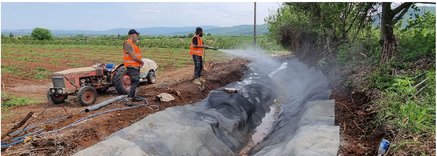
CCX-M™ hydrated after installation
