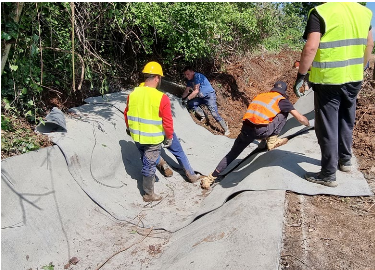
CCX-M™ laid transversely
