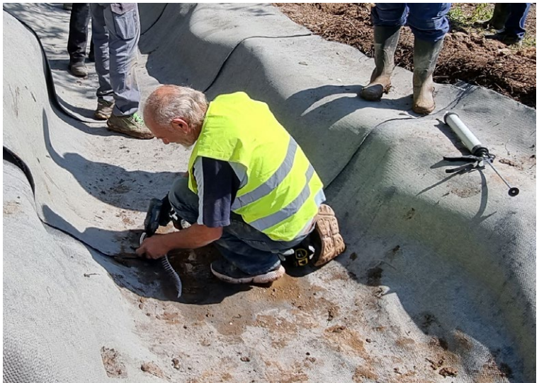
Overlapped edges secured with 30mm long screws
