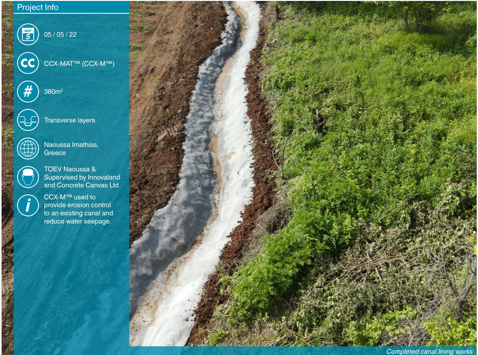
Completed canal lining works
