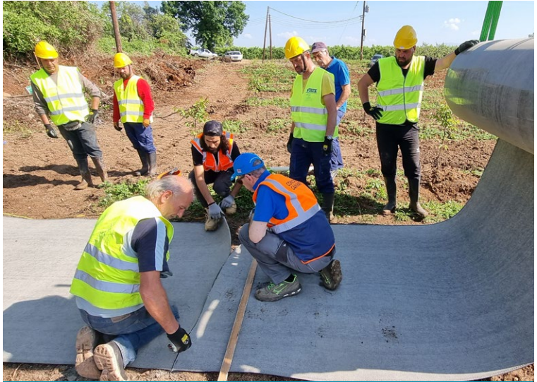
CCX-M™ rolled out and cut to desired length
