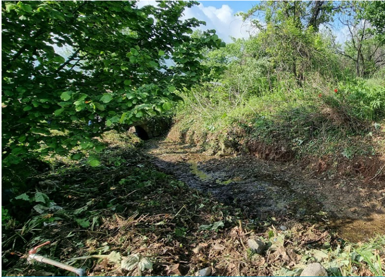
Existing canal before work commenced
